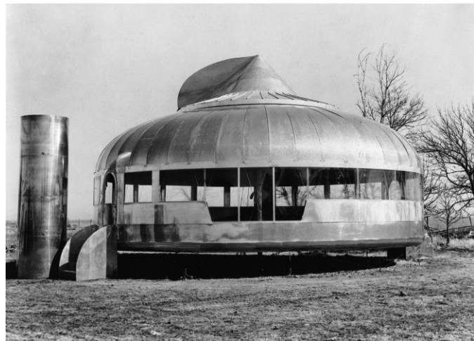
Figure 4. The Wichita House designed by B. Fuller and manufactured by an aircraft company.
