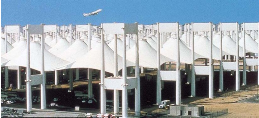
Figure 5. Teflon coated fabric roof of Jeddah Airport, Haj Terminal, UAE.
