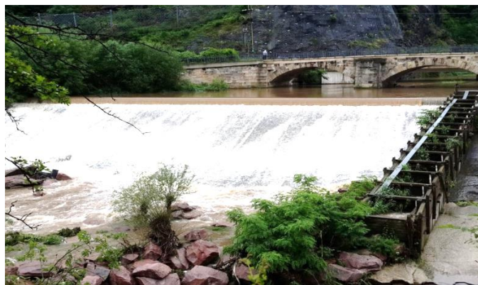
Figure 5. Vertical slot fish passage structure next to WKA Bienertmühle weir [5].
