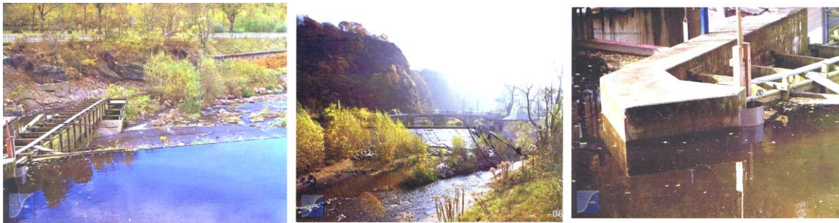
Figure 7. Plan and close-up views of potential novel fish passage at WKA Bienertmühle weir [5].
