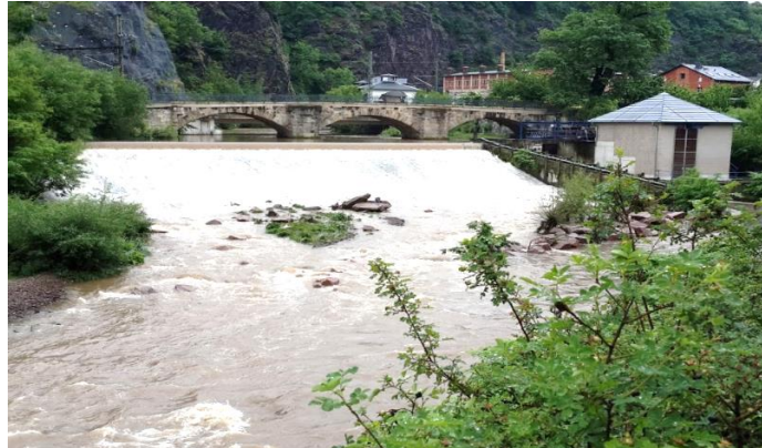
Figure 4. WKA Bienertmühle weir, fish passage and hydro power plant [5].
