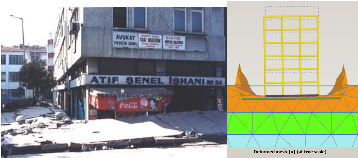
Figure 4. Example of What Happens When the Foundation Bearing Capacity of a Structure Without Basement is Exceeded [9] and Finite Element Mesh
