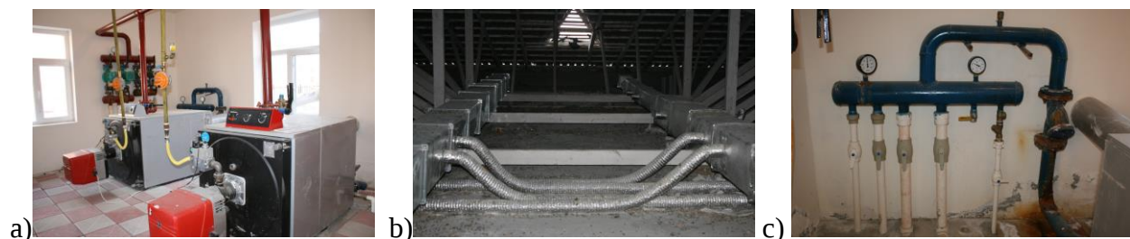
Figure 3. Energy auditing of school building: a- boiler house, b- attic with mechanical ventilation system, c- manifold of heating system in the boiler house
